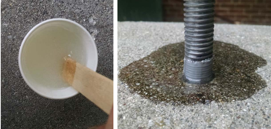
Figure 8.4 Mixed Epoxy (Left) and Installed Anchor (Right)
