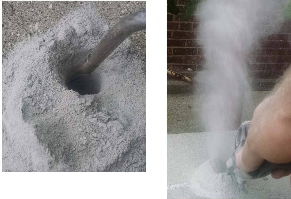
Figure 8.3 Hole Cleaning with Compressed Air
