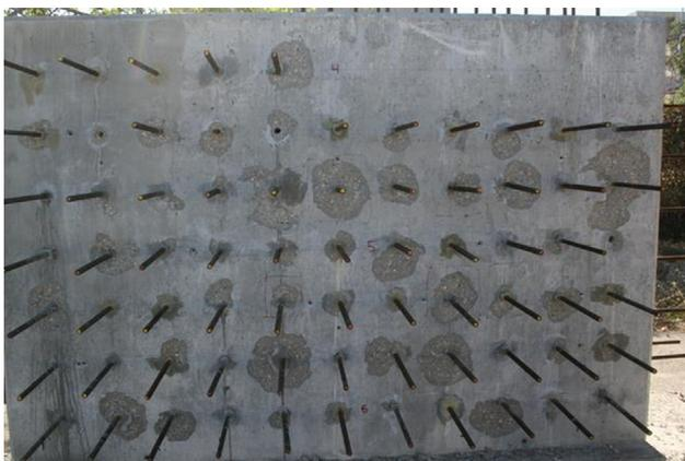
Fig. 2. The anchors drilled in one of the walls.
